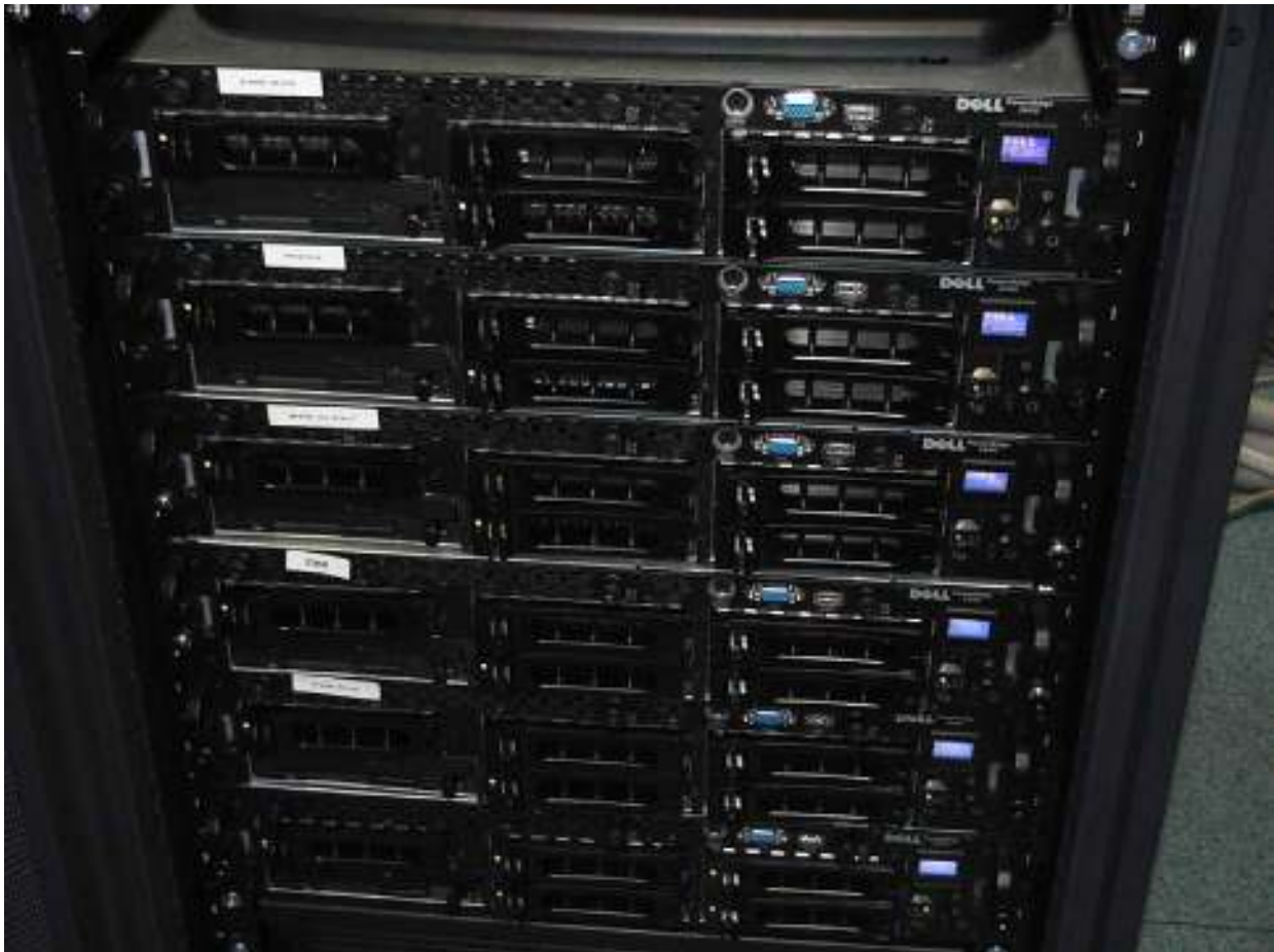
Figure 3: Dell Rack mounted servers running the EMM public and internal web servers and alert systems.
